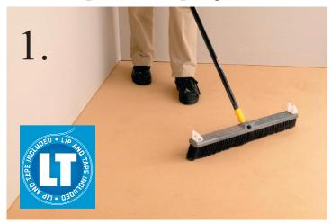
1) Subfloor surface must be clean and dry before installation.
