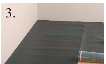
3) Roll out next row in the same manner butting foam close to first row and covering overlapping moisture barrier lip. Do not overlap foam pad just the moisture barrier lip.
