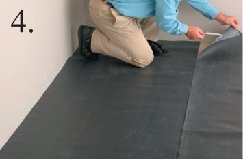
4) Remove tape liner and secure the overlapping moisture barrier to it. Continue with installation. Seal all open seams with aggressive adhesive plastic tape.
