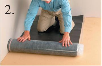
2) Start in a corner. Unroll SolidBlack HD underlayment over subfloor with vapor barrier film (Logo Imprinted Side) **down** against subfloor. Be sure tape strip side is next to the wall and overlapping lip is toward the open room.
